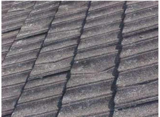
Pressed metal tiles can be dented and damaged easily over the years.
