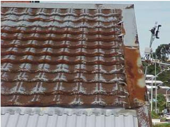
Rusted flashings can rot away completely
