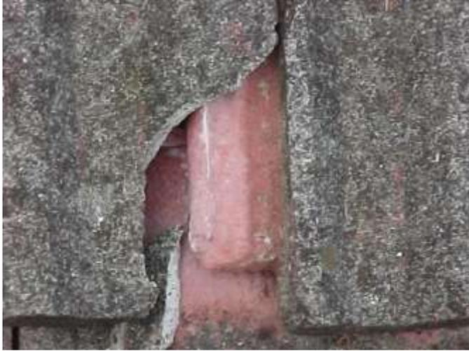
The tile surface becomes wet and during the winter when it freezes, it expands, cracking the surface, causing pits and crazing, then erosion begins. The sand and aggregate eroded from your tiles washes into your gutters. As the surface degrades, moss becomes established, it grows between the tiles and under the laps taking water directly to the timber beneath. Even a thin covering of moss is a problem, but worse still a thick covering hides the damage to the tiles.
