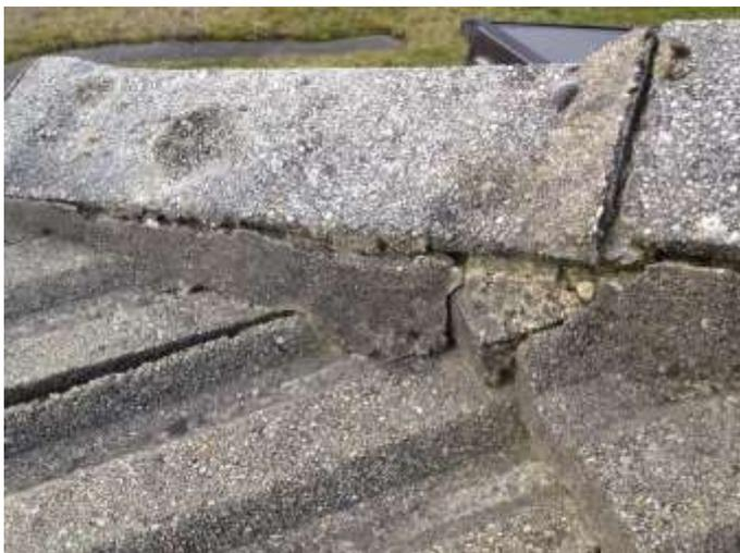
Hips and ridges can become loose and need securing so they don't blow off in the wind.
